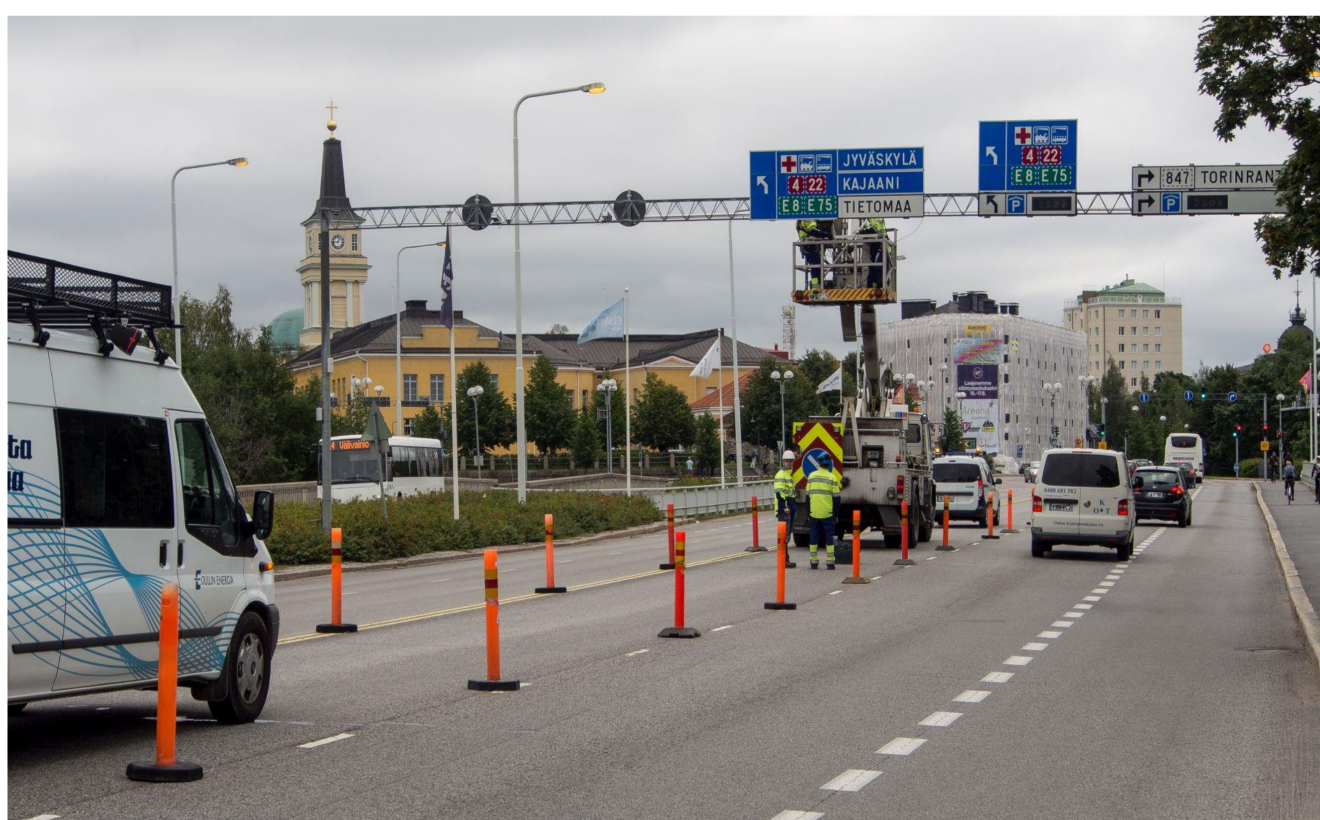
Instrument installation work onto the gantry
